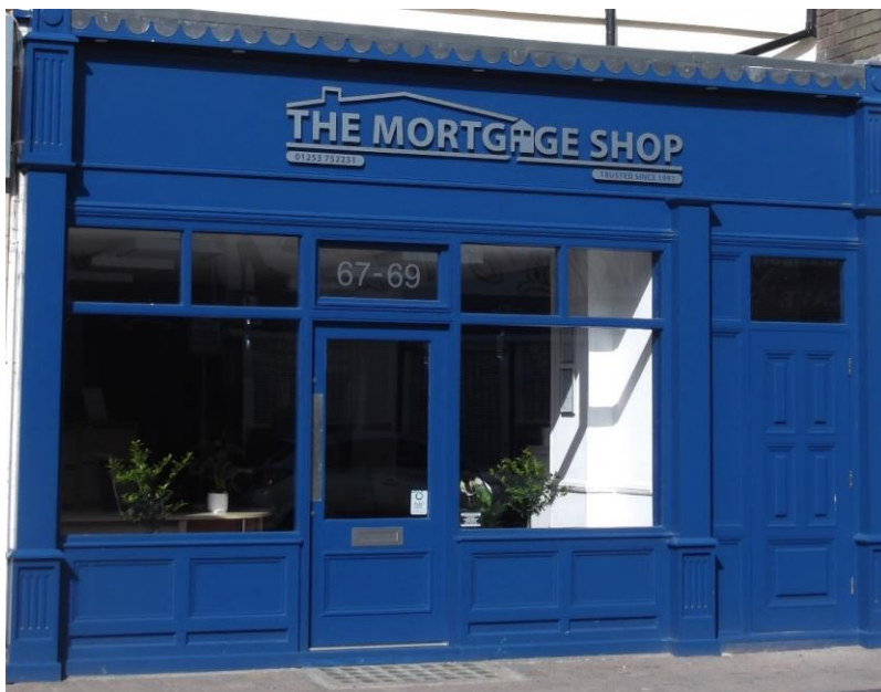
Traditionally designed shopfront
